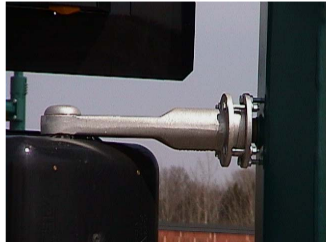
32A One-way signal mount, 45B Hub & Nipple, CAP Sealed cap. Dwg. 1A, 18, 19.
