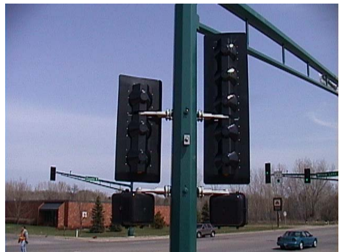
32A One-way signal mount, 45B Hub & Nipple, CAP Sealed cap. Dwg. 1A, 18, 19.
